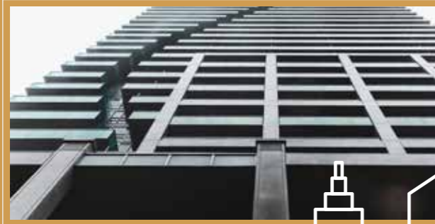
Public and private building
